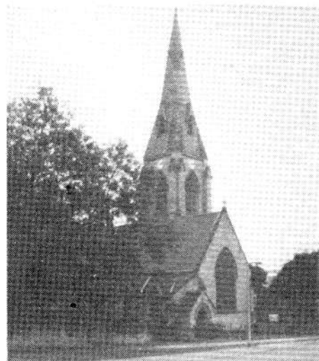
The church of St. Matthias, Burley, Leeds
