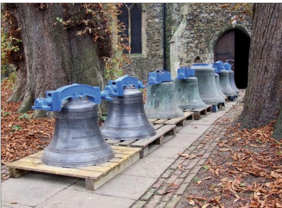
*The refurbished and augmented ring immediately before installation*
